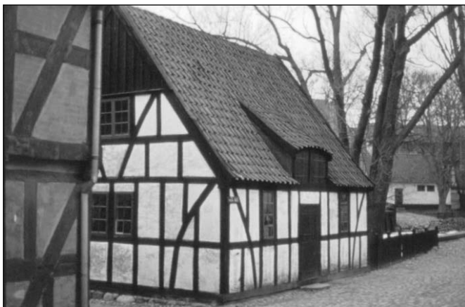
Figure 13.41: Traditional way of filling spaces with brick in a timber framed building in Denmark.
