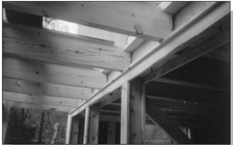
Figure 13.34: A structure designed for re-use. The structure is made of prefabricated standard monomaterial components, timber and concrete, which can easily be dismantled and re-used. Source: Gaia Lista, 1995
