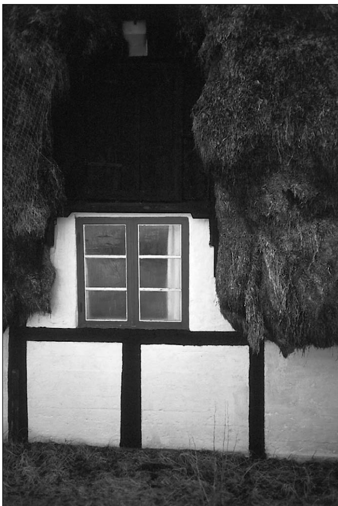
Figure 15.27: Thatching with eelgrass, Denmark.
