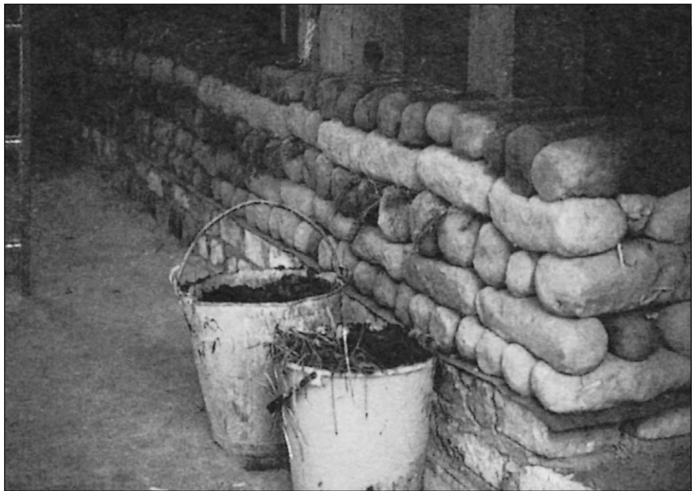
Figure 13.27: The earth loaf technique.
