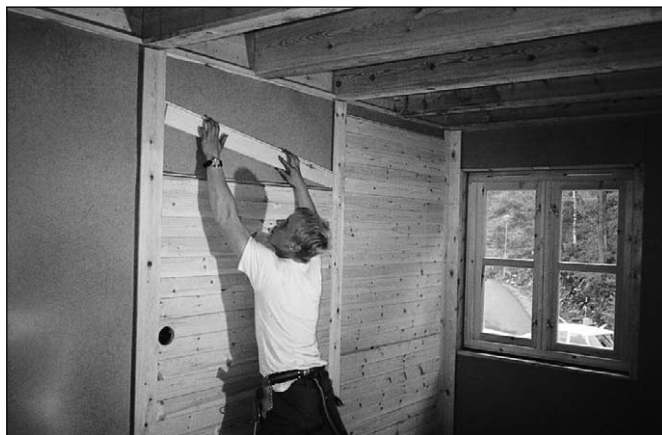
Figure 15.21: The construction of demountable internal panelling.
