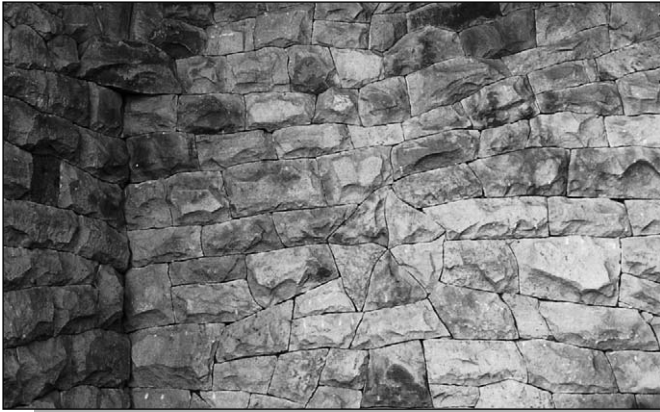
Figure 13.10: Dry-stone walling of specially cut stone.
