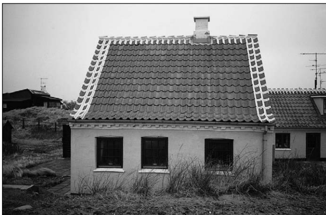
Figure 15.7: In exposed coastal areas of Denmark, the roof tiles along the ridge and the gables are fixed with lime cement mortar to prevent them blowing off.
