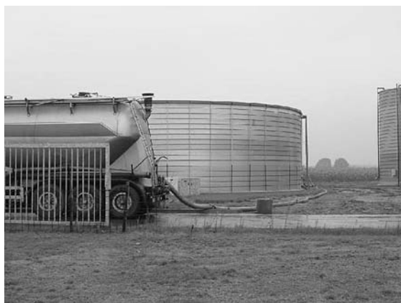
Figure 4.51 Storage tank and transportation of residue. 91)
