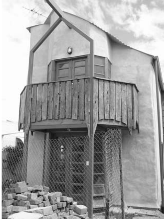
Fig. 10.1 Increasing availability and use of alternative building materials is an indication of developing sustainability. This straw-bale cottage is one of four being constructed alongside concrete block apartments. The buildings are part of the 'Christies Walk' Eco-City development in inner-city Adelaide developed in association with the UN registered non-government organisation, Urban Ecology Australia.
