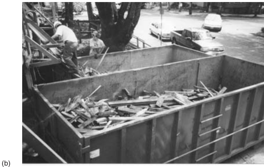
Fig. 3.15 Construction and demolition waste and job-site recycling. (a) Unsorted construction debris on a commercial building project in Singapore becomes a burden on scarce landfill sites. Photograph courtesy of undergraduate construction management student, Department of Building and Construction Economics, RMIT University, Australia. (b) On-site separation of waste streams for recycling can save money as well as divert materials from landfill. Here timber from a house deconstruction project in Oregon, USA, is sorted into a bin for recycling. Photograph courtesy of the Centre for Building and the Environment, R.E. Rinker School of Building Construction, University of Florida, USA.
