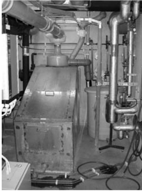
Fig. 11.6 Aquatron, urine separator and composting toilet unit. Architect: White Arkitekter AB. Photograph by Tomas Lexén.
