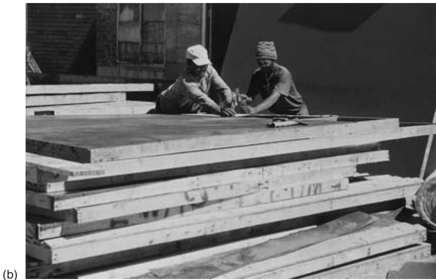
Fig. 3.12 People in developing countries can't afford to waste resources. (a) Recycling yard in the Cape Flats area, Cape Town, S.A. (b) Prefabrication in the Cape Flats area, Cape Town S.A. These wall frames are made from salvaged timber and metal sheet and, for those who can afford them, become the walls of 'informal' dwellings in sprawling squatter settlements.
