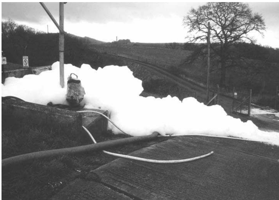
Fig. 32.5 A biological (nocardioform) foam similar in appearance to a detergent foam.
