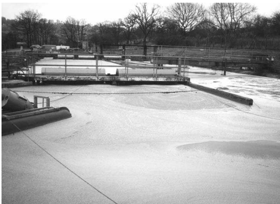
Fig. 32.6 Foam can be managed to an acceptable level and retained on the surface of the aeration tank.
