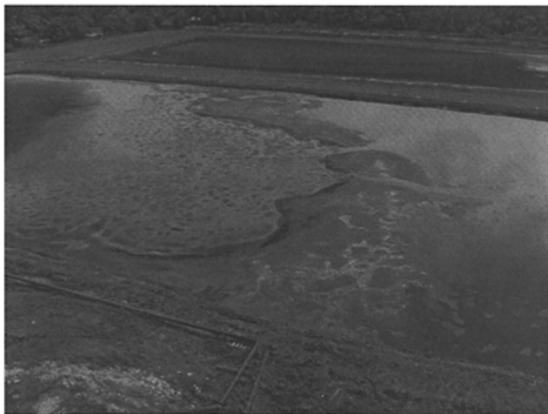
Figure 6 Formation of islets of sludge in the middle of the pond. (Courtesy of Felda Palm Industries.)
