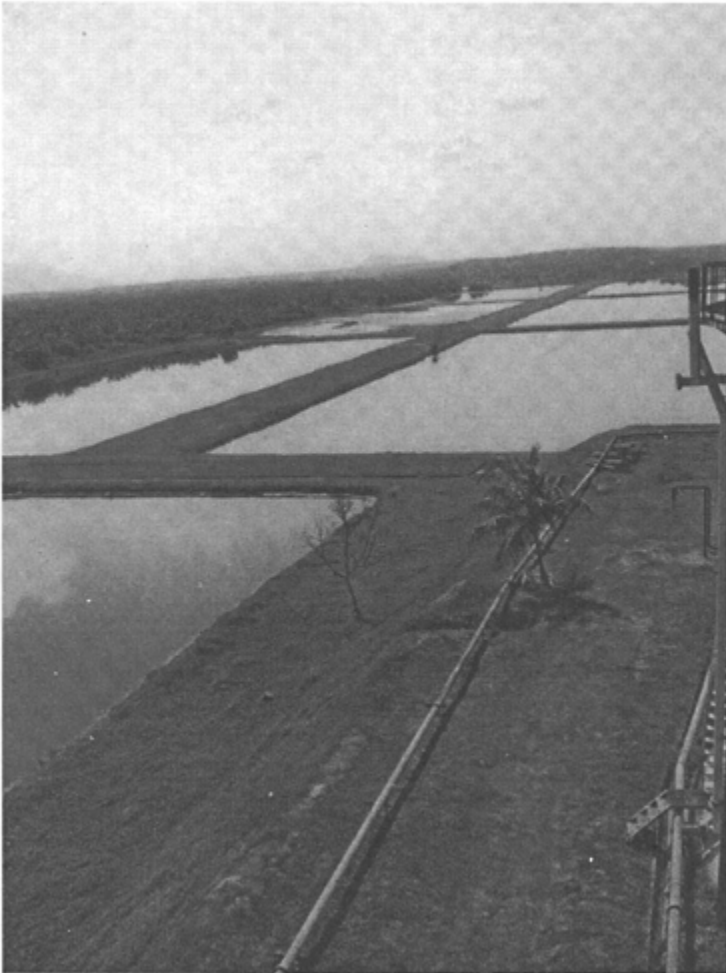
Figure 4 A series of ponds for POME treatment occupying a large land area. (Courtesy of Felda Palm Industries.)
