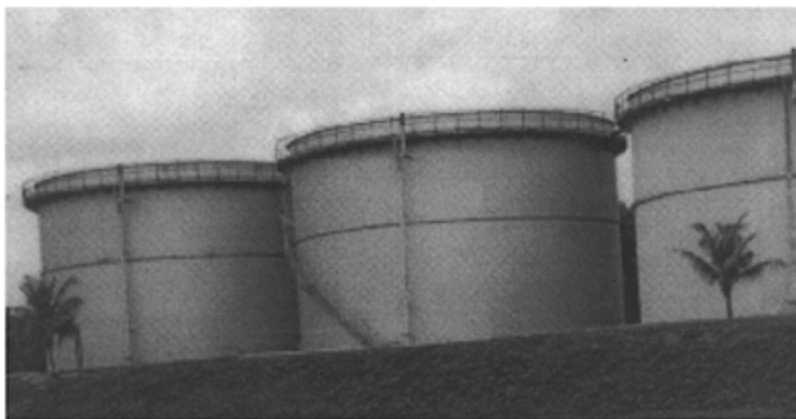
Figure 7 A series of 3600 m 3 open digesters for POME treatment. (Courtesy of Felda Palm Industries.)
