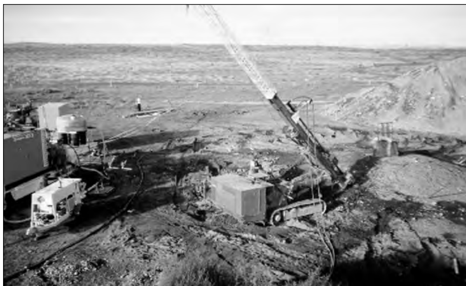
Figure 1. Casa Grande jet grouting unit used for in situ stabilization of pit G-11 at Brookhaven National Laboratory.
