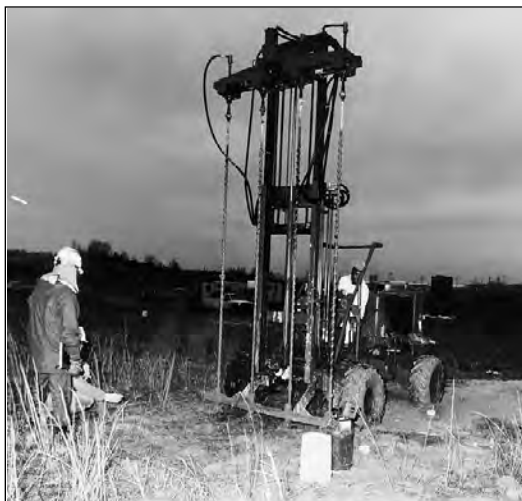
Figure 2. The HBE multipoint injection system during field trials at the DOE Portsmouth Plant.
