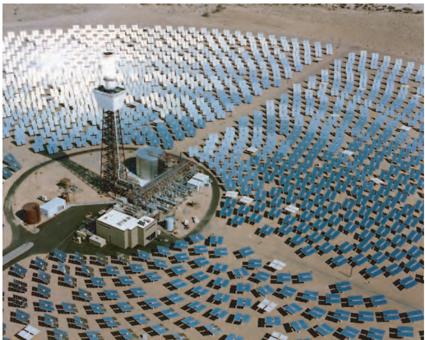
Figure 8.4. Reflectors focusing solar energy onto a 10-megawatt receiver power tower, called Solar One, in Barstow, California. Photo by Sandia National Laboratory Staff, available from the National Renewable Energy Laboratory.
