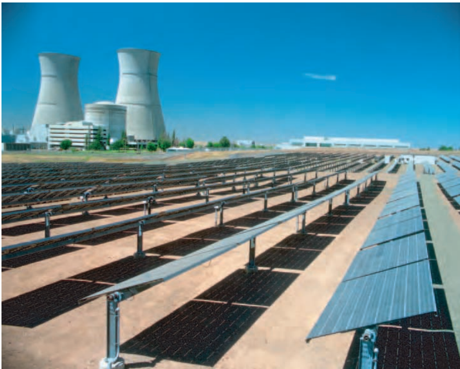
Figure 8.6. Solar photovoltaic system colocated with a nuclear power plant at the Sacramento Municipal Utility District's Rancho Seco facility. The photovoltaic system (2 megawatts), spread over 8,094 m 2 , produces power for 660 homes. Photo by Warren Gretz, available from the National Renewable Energy Laboratory.
