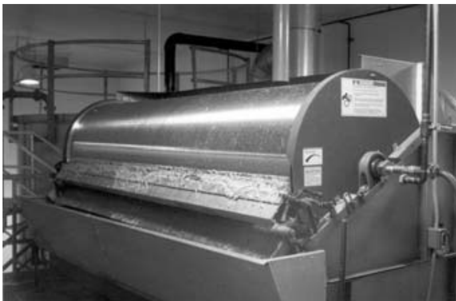
Figure 8-61 Rotating cylindrical screen. (Courtesy of Hycor.)
