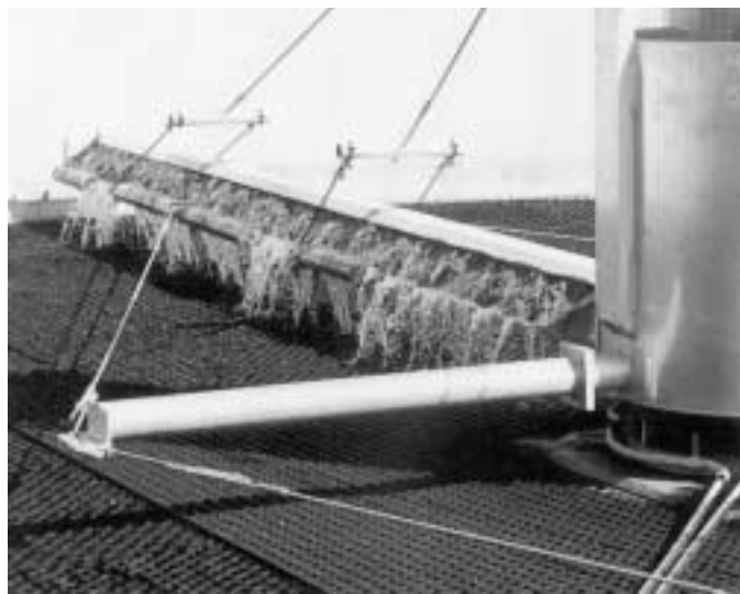
Figure 8-47 Photograph of rotary distributor for trickling filter. (Courtesy of U.S. Filter/General Filter.)
