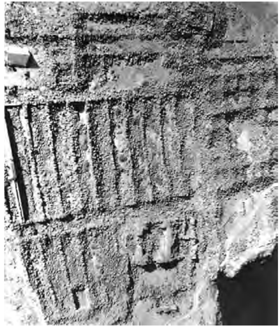
Figure 5 This picture, taken before the reconstruction of Masada, shows how the walls of the parallel storerooms collapsed into the adjacent rooms, leaving rows of bricks that are diagnostic of earthquake collapse. From Masada: Herod's Fortress and Zealot's Last Stand by Yigael Yadin, © 1966 by Yigael Yadin. Used by permission of Random House, Inc.
