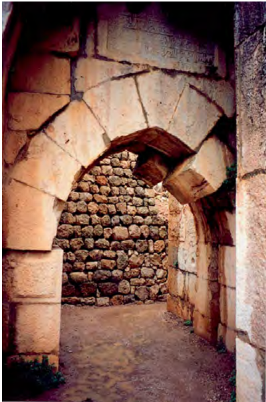
Figure 8 This is an example of a slipped voussoir in the Crusader fortification of Kala'at Namrud. Note how base of one side of the arch slipped outward, allowing the voussoir to drop.
